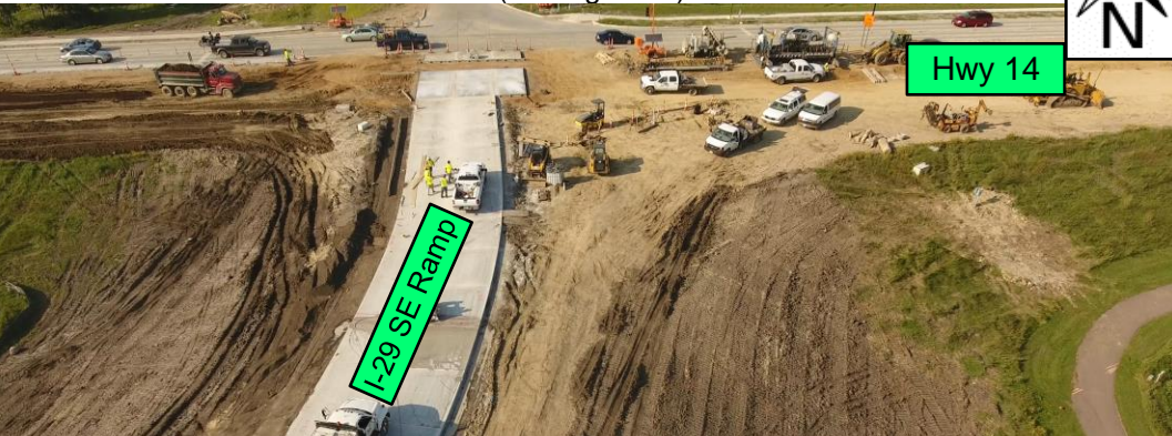
Project Photo: Work on the I-29 SE Ramp @ Hwy 14 (looking north)
