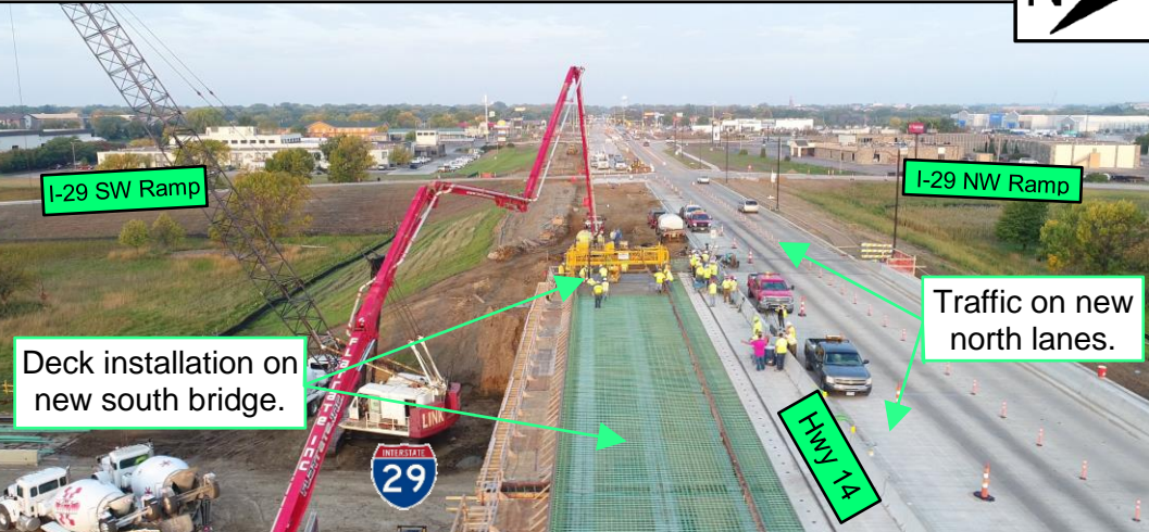
Project Photo: Work on the south bridge @ Hwy 14 (looking west)
