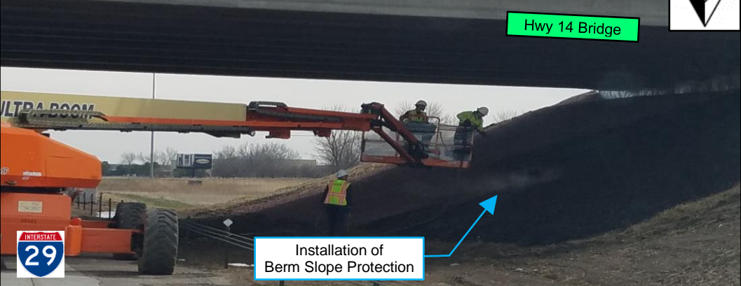
Project Photo: Project work @ I-29 @ Hwy 14 Bridge (looking south)
