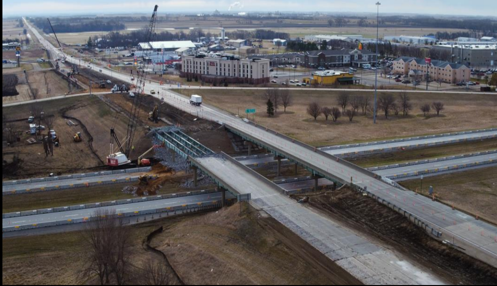
Project Photo: Bridge and pavement removals @ I-29 (looking southeast)
