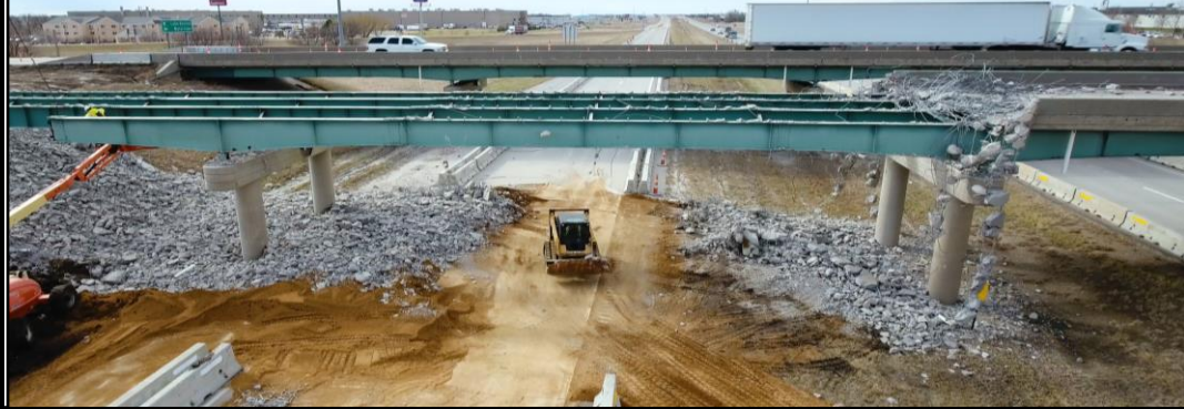
Project Photo: Bridge removals @ I-29 (looking south)
