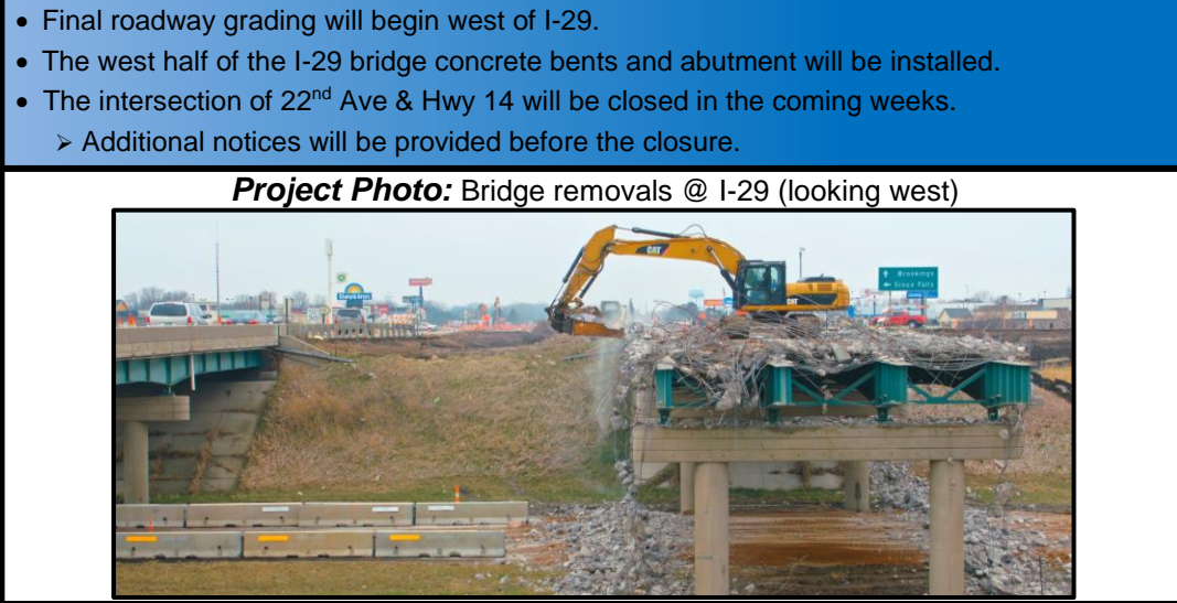
Project Photo: Bridge removals @ I-29 (looking west)
